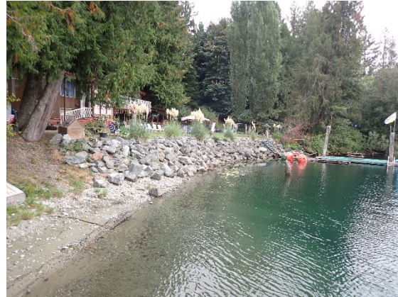
Photo 4: Riprap and fill
